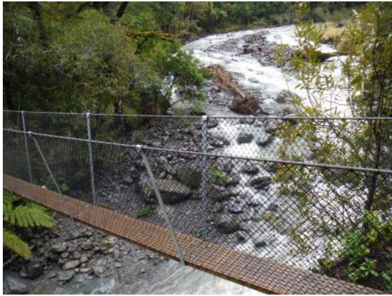
New bridge across Totara Stream
